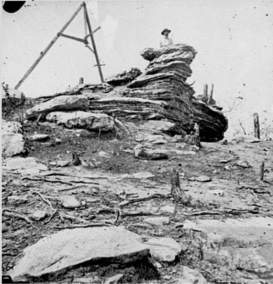
Chattanooga, Tenn., vicinity. Tripod signal erected by Cpts. Dorr and Donn of U.S. Coast Survey at Pulpit Rock on Lookout Mountain
